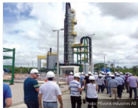
Plant for conversion of biogas from domestic waste into biomethane
