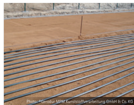
Installation of the heat-exchanger
