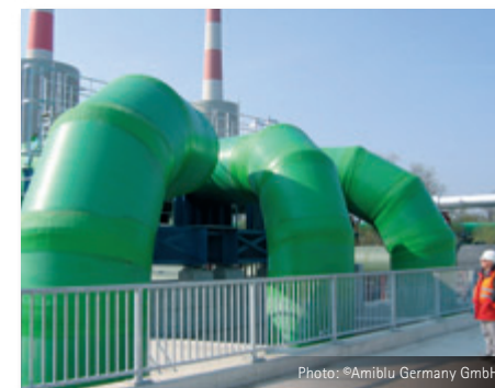
GRP cooling-water line in a gas-fired power plant
