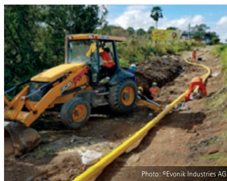
Polyamide (PA-U12) pressure lines, dimensions: external diameter 160, SDR 11
