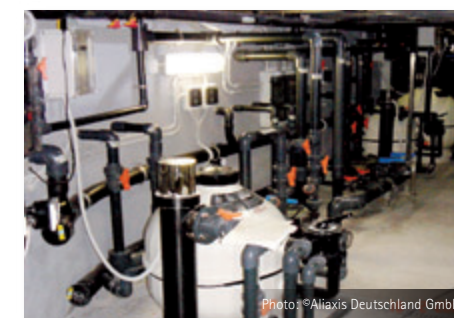
Desalination plant showing PE100 pipes and fittings
