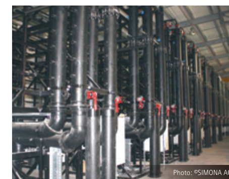
Desalination plant showing PE100 pipes and fittings
