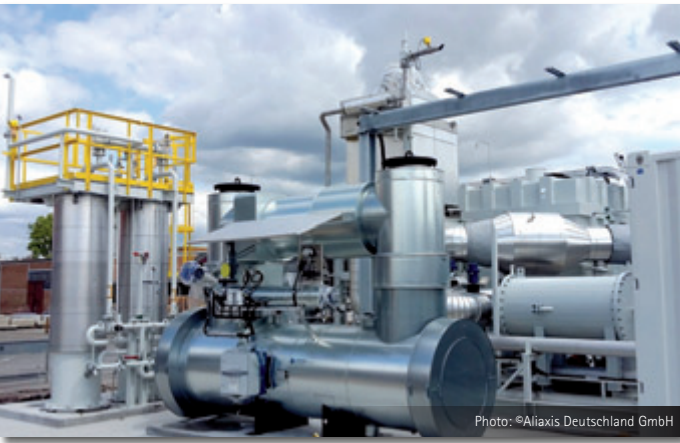
1.4 Megawatt fuel cell (MCFC) supplying energy to the production location
