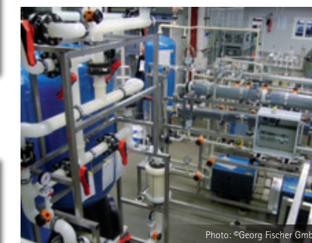
Desalination plant showing PE100 pipes and fittings
